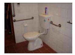
The toilet is right hand transfer with 300mm between the toilet and the nearest object (the wall). The distance from the front of the seat to the rear is 730mm and the height of the seat is 470mm. There is horizontal side and rear grab rails at 800mm height and a side vertical grab rail 950-1550mm height.
